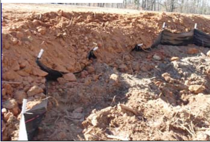
Poor general housekeeping. Lack of silt fence maintenance
