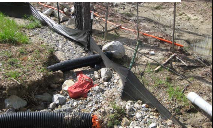
Poor general housekeeping. Lack of silt fence maintenance
