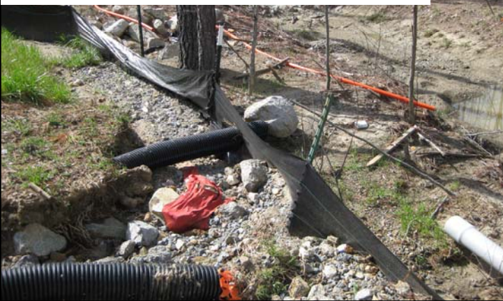
Poor general housekeeping. Lack of silt fence maintenance
