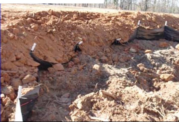
Poor general housekeeping. Lack of silt fence maintenance
