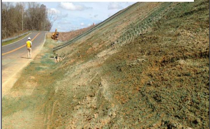
Too little mulch. Steep slopes require 3500 lbs. of mulch per acre.
