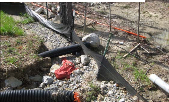
Poor general housekeeping. Lack of silt fence maintenance
