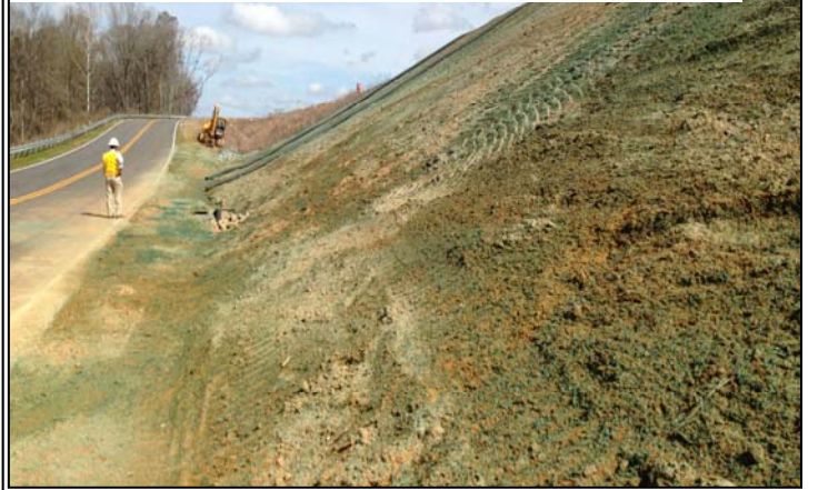
Too little mulch. Steep slopes require 3500 lbs. of mulch per acre.
