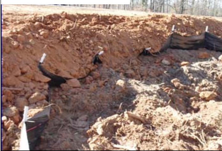
Poor general housekeeping. Lack of silt fence maintenance
