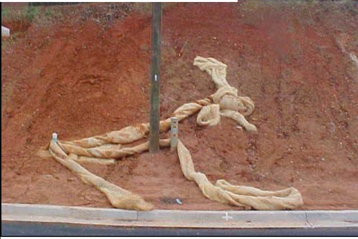
Too little mulch. Steep slopes require 3500 lbs. of mulch per acre.
