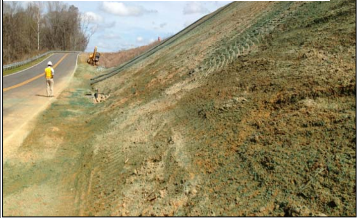
Too little mulch. Steep slopes require 3500 lbs. of mulch per acre.
