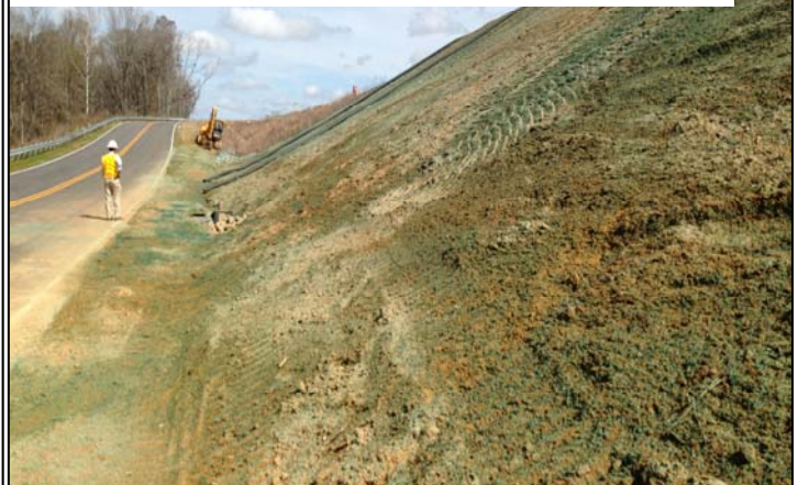
Too little mulch. Steep slopes require 3500 lbs. of mulch per acre.
