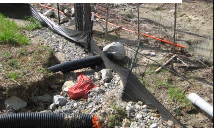
Poor general housekeeping. Lack of silt fence maintenance
