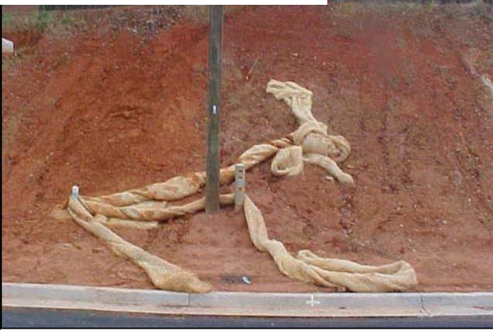
Too little mulch. Steep slopes require 3500 lbs. of mulch per acre.
