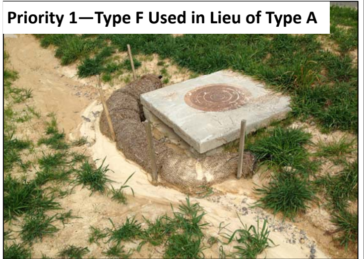
Priority 1—Failure
