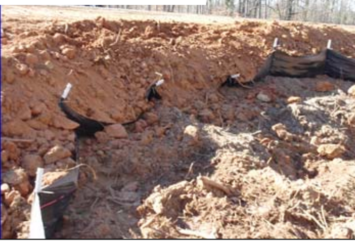
Poor general housekeeping. Lack of silt fence maintenance
