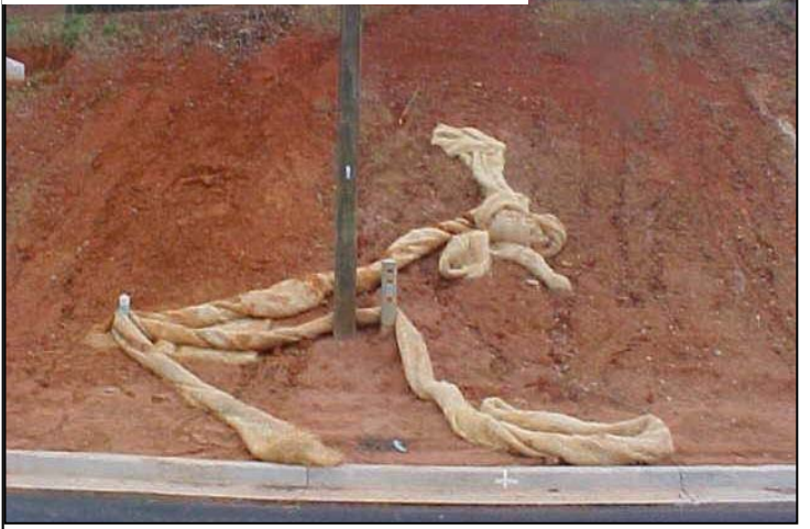
Too little mulch. Steep slopes require 3500 lbs. of mulch per acre.
